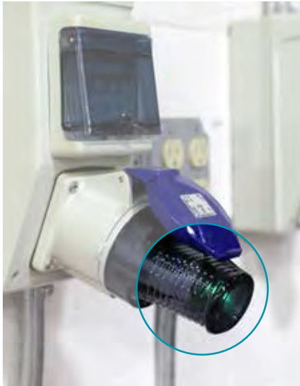
GREEN LAMP LIGHTS Phase sequence is correct
